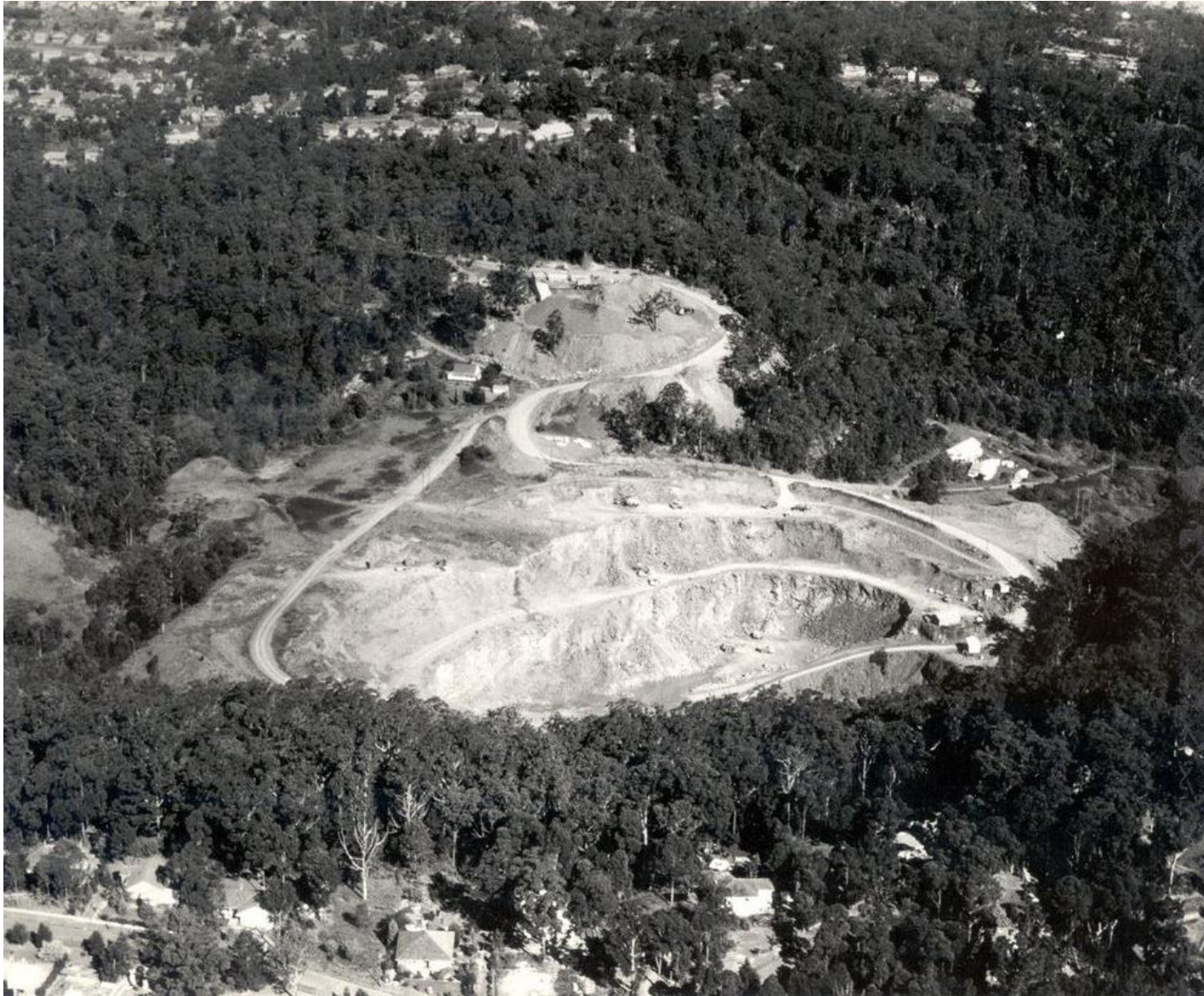
Figure 2. 8 Aerial view looking South towards Crusher Plant early 1960s
